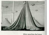
part of the top ring, the ring is lifted and the fabric unfolds, [6.3.13] The principles of the construction process are illustrated in this perspective sketches of a corner unit.
