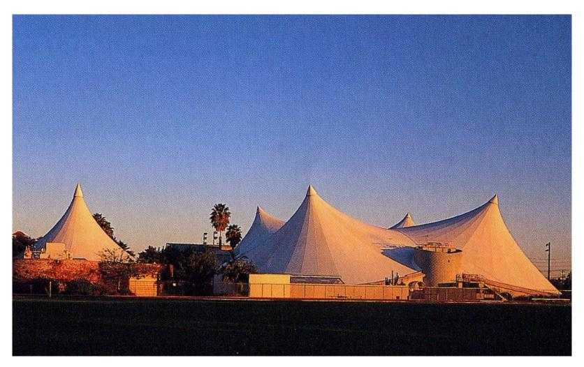
One of the first architectural applications of PTFE coated Fibreglass fabrics developed in 1972. Fabric was tensile tested after 20 years at 70% fill/80% warp of original strength.
