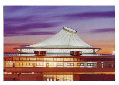
Membrane Structures are optimized for structural live loads and are designed with a specified prestress, which affects the equilibrium shape. Support conditions, membrane stiffness, and biaxial properties are also factors in the final form.
