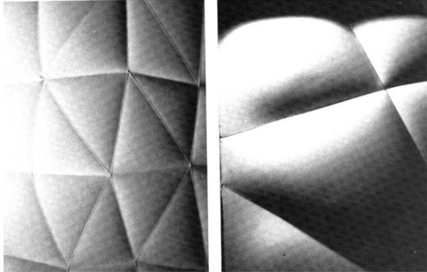
Above: Lost fabric formwork for poured earth.
