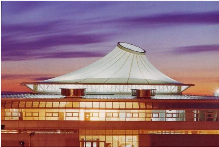
Membrane Structures are optimized for structural live loads and are designed with a specified prestress, which affects the equilibrium shape. Support conditions, membrane stiffness, and biaxial properties are also factors in the final form.
